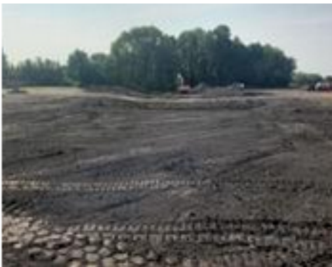
During Construction: Berm and installing tile at head of gully
