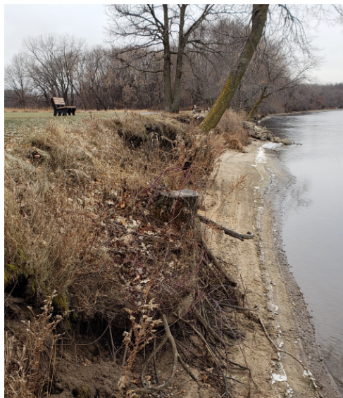
Project area prior to construction.
