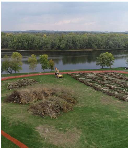
Staging of material before the start of the project.
