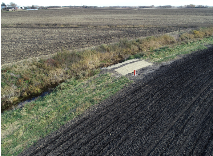
After: Side inlet installed in late September.
