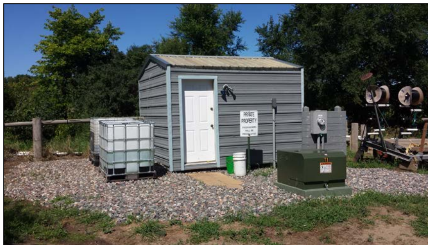
This shed controls the Marties' SDI system
