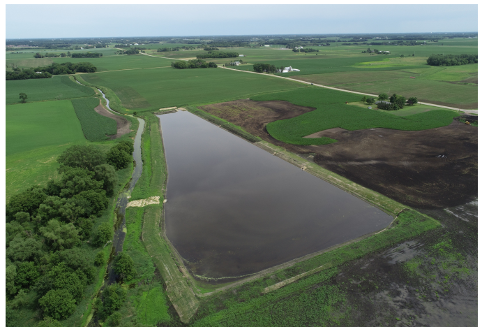
Sediment Pond vegetation established in August.
