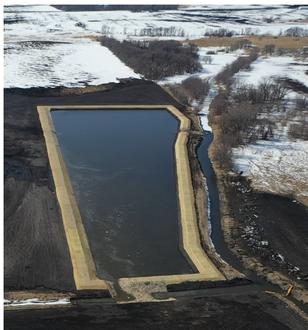
Completed Sediment Pond in early March.
