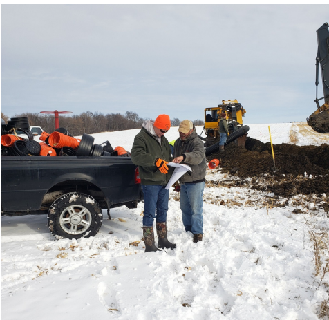
District Manager Luke Johnson communicating with a contractor on construction plans.
