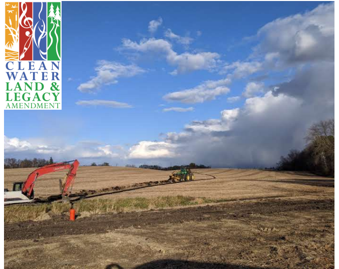
Tile being installed for seven water and sediment control basins.
