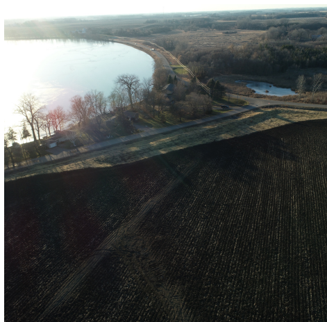
Water and sediment control basin installed on the north side of Howard Lake.
