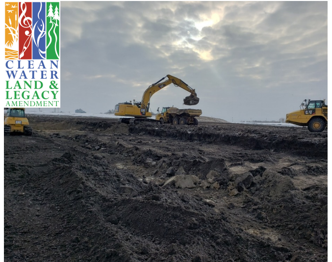
Starting to dig for the County Ditch 10 Sediment Pond.
