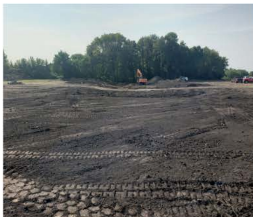
During Constructing: Berm and installing tile at head of gully.
