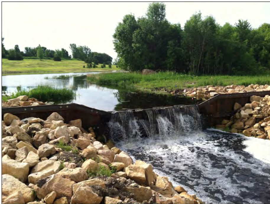
Figure 4: Sheet Pile Weir used in a Wetland Restoration
