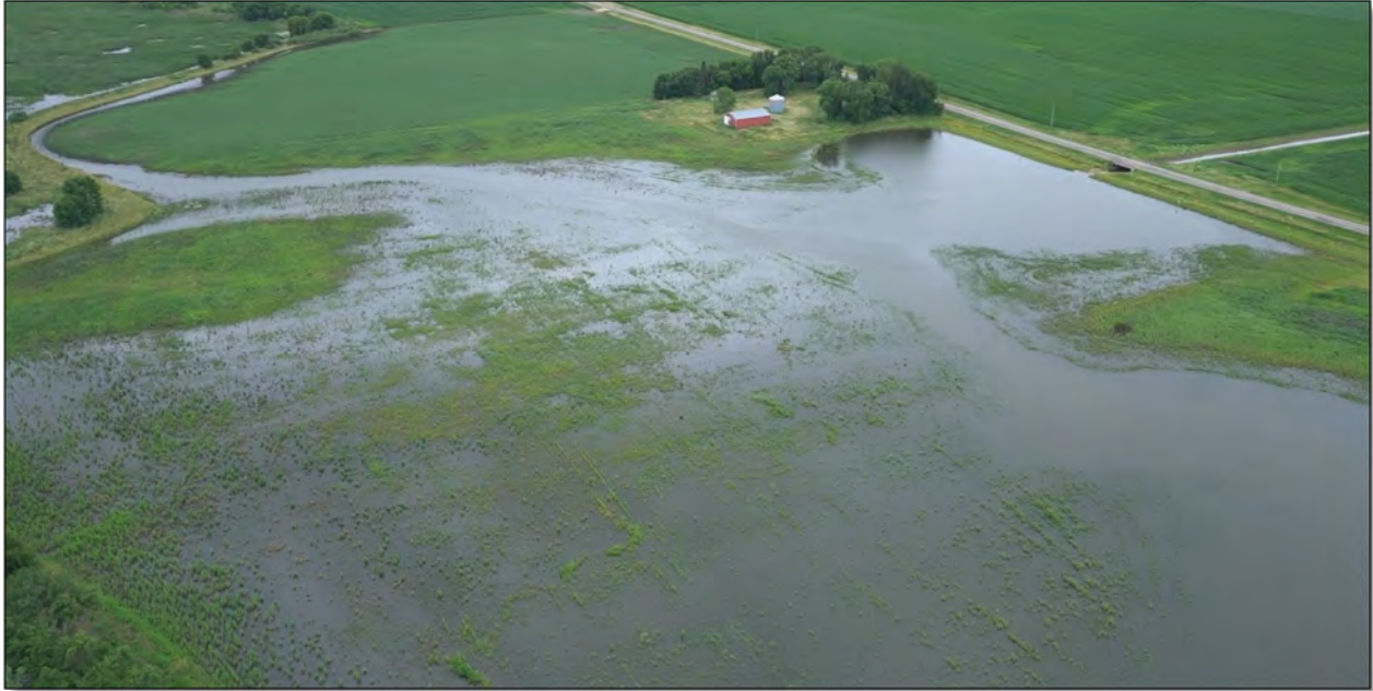
Figure 15: Storage Treatment Basin
