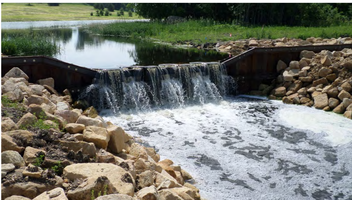
Figure 50. Wetland Enhancement Created by Weir Addition
