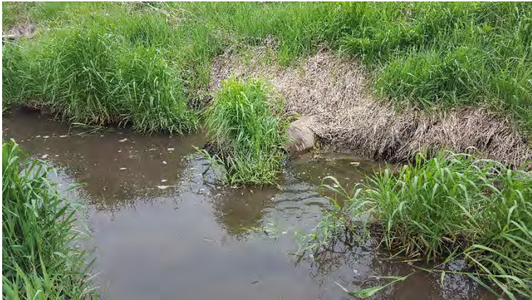
Figure 41. Covered Tile Outlet Draining into Main Open Ditch.
