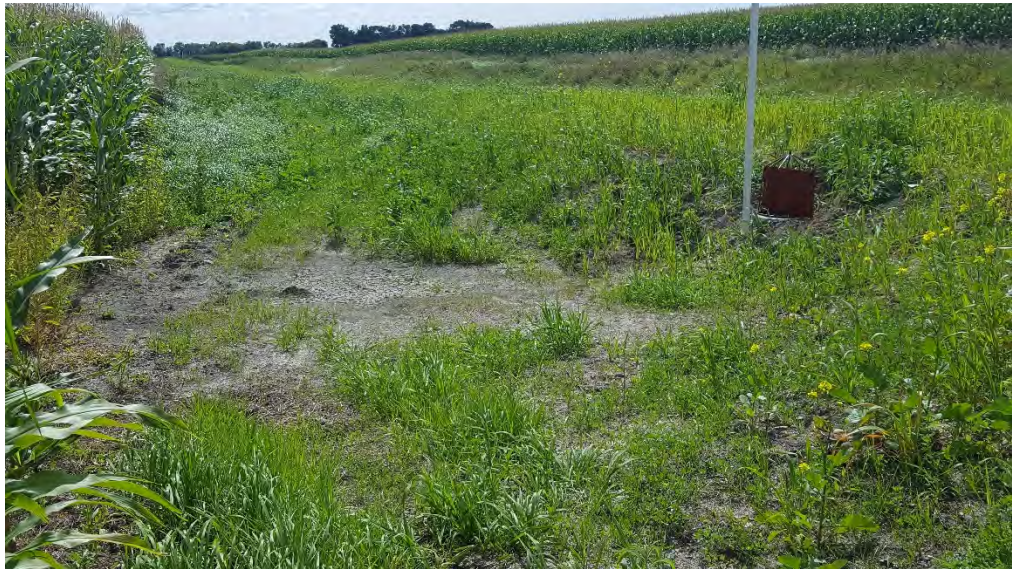
Figure 47. Typical Constructed Side Intake
