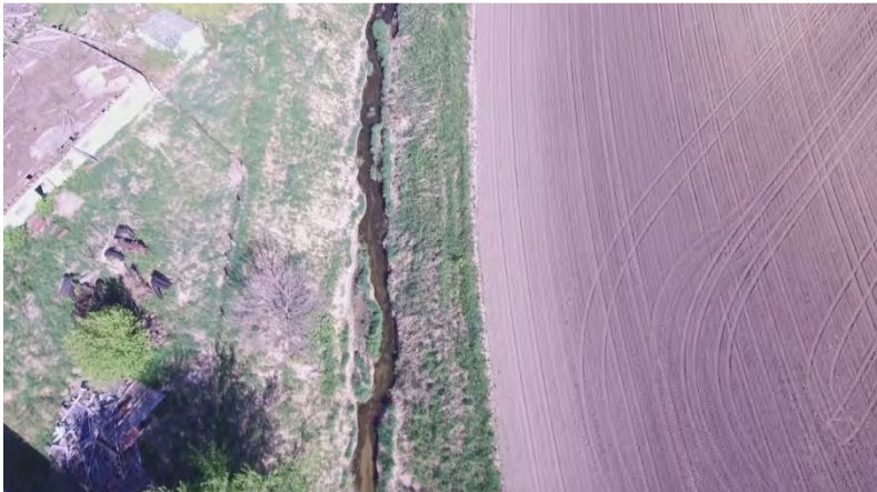
Figure 33. Sloughing along open ditch in Northeast Quarter of Section 24 in Stockholm Township on Sieg Lateral
