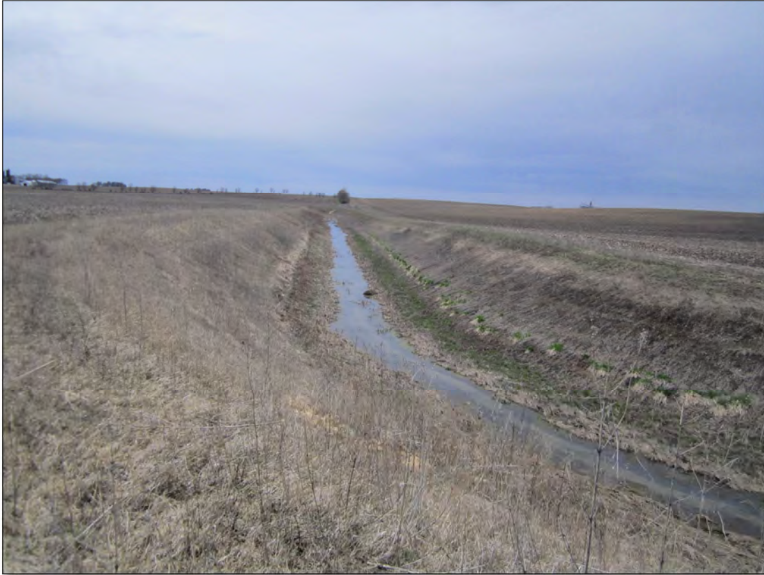
Figure 5: Two-Stage Ditch Constructed in Blue Earth County
